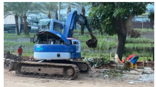
Construction works are conducted as usual.
